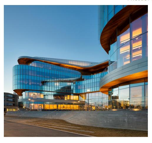
The Tropical Forest Products Rain Screen and Soffit System is an engineered system in which all of the design components play an interdependent role in the system's performance. Each installed system is stamped and certified by a licensed state engineer to comply with state building code wind load compliance requirements.
