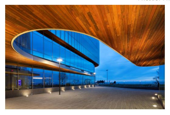
The Kellogg Global Hub design team's solution was to use an innovative system to attach the wood soffit: the Tropical Forest Products Rain Screen and Soffit System.
