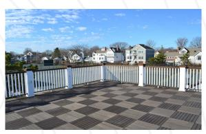
Tropical Forest Products Deck Tiles are Ideal for poorly ventilated deck applications. Material and labor costs are lowered significantly when using modular deck panels.
