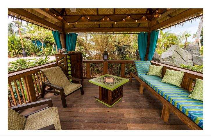
Cumaru was recently selected for cabana and bridge decks, stair treads and rails for Universal Studios Volcano Bay Water Park. Of interest was the determination during the design phase of the project, that when tested, smooth surface Cumaru had a higher dynamic coefficient (slip resistance) than grooved decking profiles, despite the perception of being (non-slip). Smooth decking creates more contact area between the sole of a shoe and the deck surface then grooved decking.
