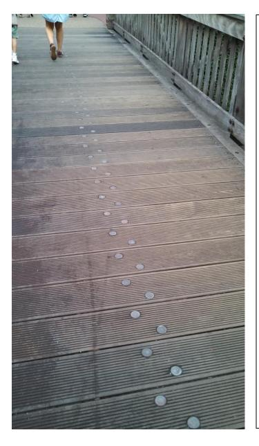
Naturally resistant to anything nature can throw at it as well as the daily cleanings and the millions of visitors it supports, Ipe remains the gold standard for commercial and residential exterior construction Projects. Note the unique grooved decking profile and fastening system developed by WDW for this bridge deck application.
